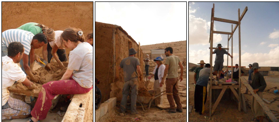
Left: Mixing mud and straw render; Middle: The new khan at Qasr As-Sir; Right: The beginnings of a new compost toilet (#4 by Bustan Qaraaqa). Thanks to Allison for these pictures!
